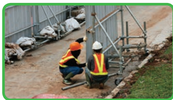
• November 2013 , Preparation for underground construction along Senayan-Bundaran HI corridor.
